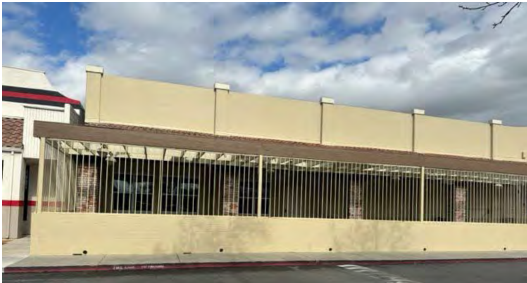
Figure 4 – Existing Garden Center
